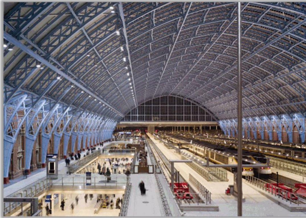
Figure 4: St Pancras International Railway Station 32
