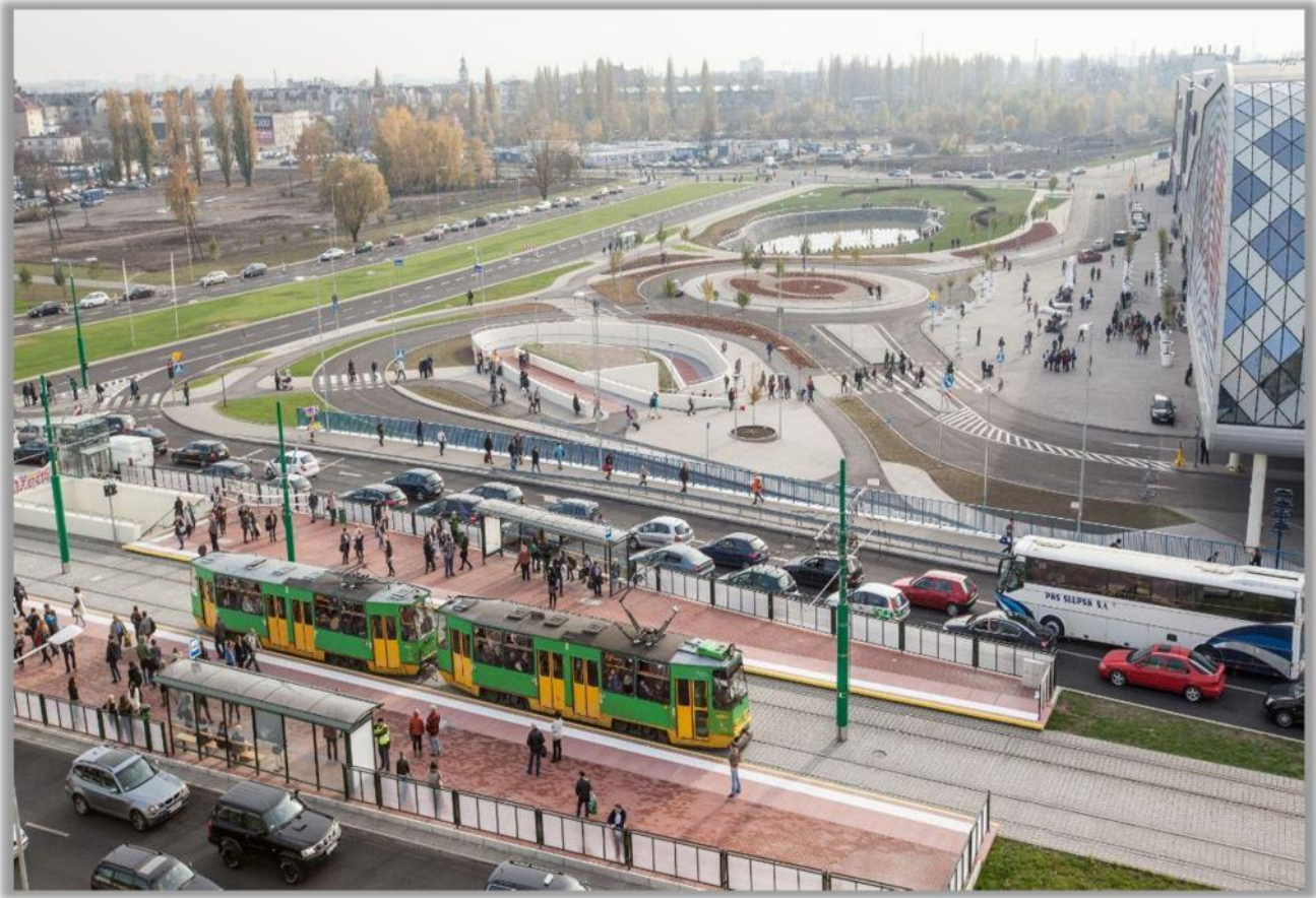
Figure 8: The new station provides better transfer between multiple modes of transportation and incorporates many mitigation/runoff features 60
